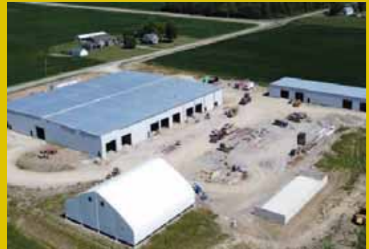
Wells County Highway Garage
