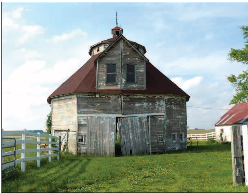
The Rudicel-Montgomery Barn near Waldron in Shelby County is a unique 12-sided barn that was built in 1910. It was part of the Indiana Barn Foundation's Barn Tour on Saturday, Sept. 14. (Photo by C.J. Miller)
