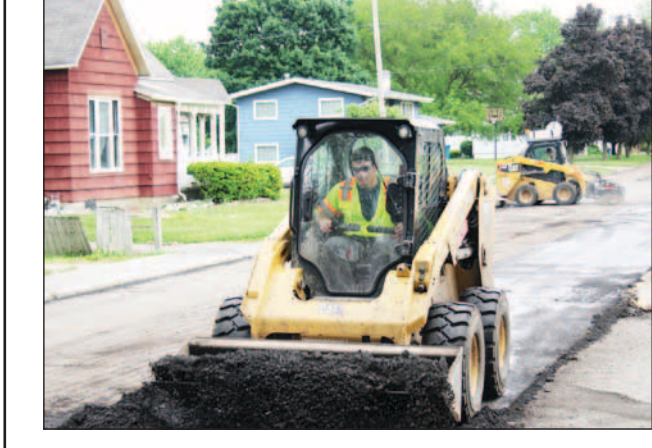
Roadway Refresh ADA curb work is mostly completed for the construction crews, so the milling and paving process has begun in Bluffton. The milling work, which removes the surface of a road so paving crews don't elevate the roadway, is currently being done on Silver Street pictured. Crews are currently working on Townley Street, with Horton Street's paving close to completion. (Photos by Jonathan Snyder)
