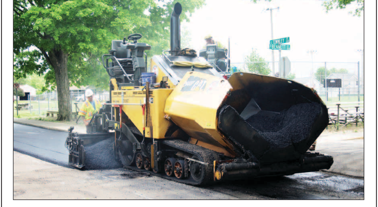
Roadway Refresh ADA curb work is mostly completed for the construction crews, so the milling and paving process has begun in Bluffton. The milling work, which removes the surface of a road so paving crews don't elevate the roadway, is currently being done on Silver Street pictured. Crews are currently working on Townley Street, with Horton Street's paving close to completion. (Photos by Jonathan Snyder)
