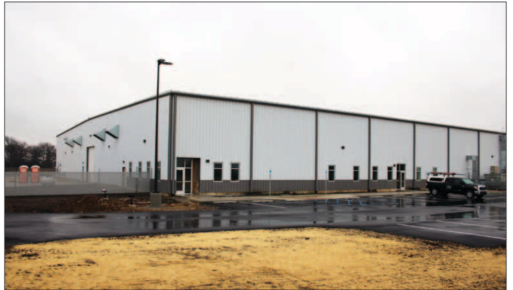
The site for the new highway building is located at 0828 E 200 S in Bluffton. The project will be completed in February. (Photo by Holly Gaskill)
