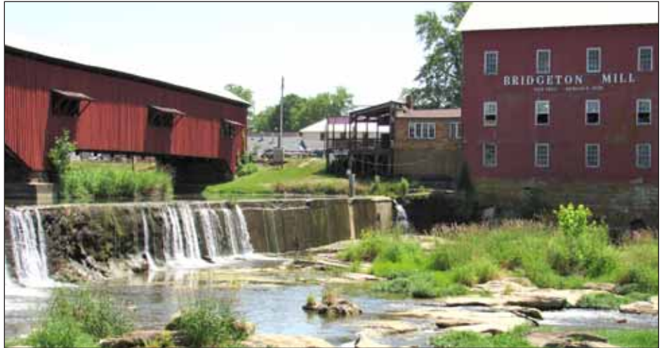
Probably the most famous of Parke County's 31 covered bridges is the 245-foot-long bridge at Bridgeton (at left in above photo). It burned down twice, the last time in 2005 was believed to be arson. (Photos by Rod King)
