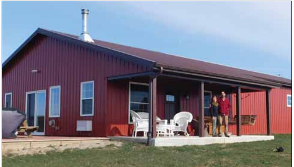
LaNae and John Abnet got rid of most of their possessions, literally measured what was left, and built walls to fit when they constructed a 750-square-foot home on 32 acres of prairie and woods west of Geneva last year. Their attached garage is much larger than their one-room living space. (Photo by Tanya Isch Caylor)
